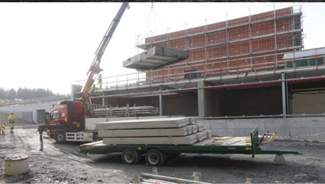
POP UP Concrete prefabrication factory – on site
