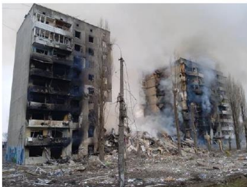
The town of Borodyanka, Kyiv oblast. The bombardment has cut the residential building in half.
