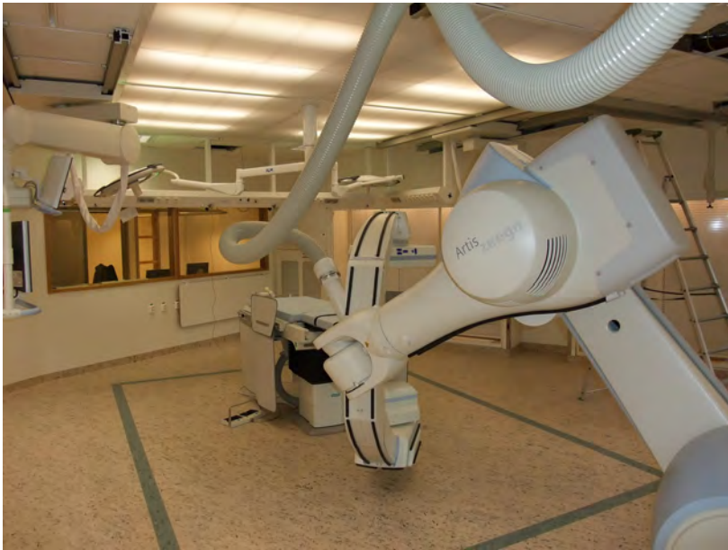
Fig. 15. Example for a Laminar Airflow ceiling ensuring a clean environment above the surgical area
